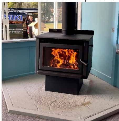
Our new wood-burner fireplace
