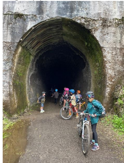
The abandoned tunnel- riding into the dark was a challenge
